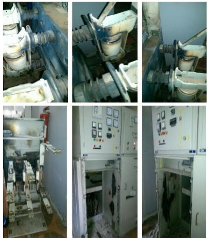
**Fig.7.** Explosion of the Expansion Chambers Effects
