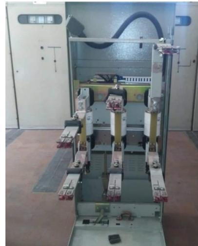
**Fig.4.** The circuit breaker (SF<sub>6</sub>).
