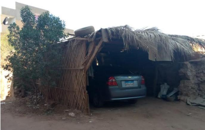
Figure 9 A garage made from prefabricated date palm midribs panels in Dakhla oasis.
