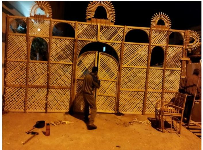
Figure 10 A timber framed date palm midribs fence in Dakhla oasis
