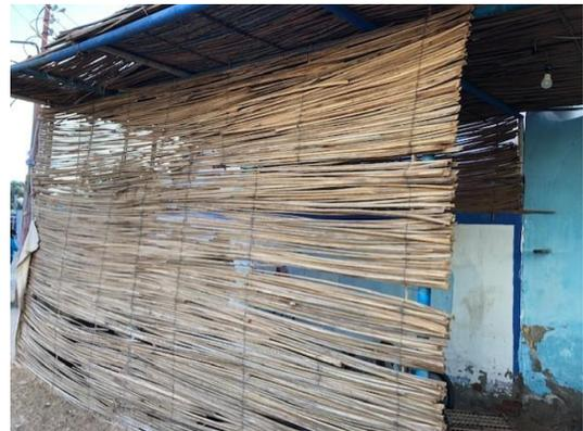
Figure 11 A steel wire-threaded date palm midribs partition in Aswan.
